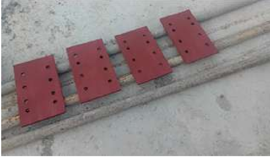
FIGURE 10. Base plate prepared for installation as per structural design and as-built drawings
