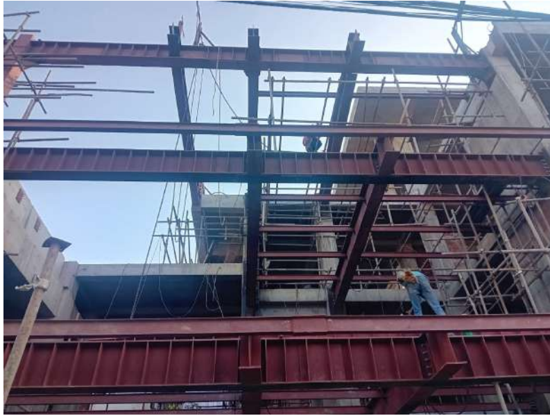
FIGURE 3. Erection of PEB 600 beam section in G+1 and G+2 floor level
